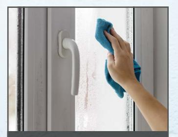
"Condensation damp" is caused by an excess of moisture in the air and poor ventilation. This causes water droplets to form on cold surfaces such as windows and walls. The risk of condensation forming is increased through daily living activities such as bathing, cooking and drying clothes. This type of damp can cause mould to form on the affected surfaces.
