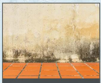
"Rising damp" happens when moisture travels up from the ground, usually on the bottom floor of a property, this is caused by defects in the foundations of the building.
